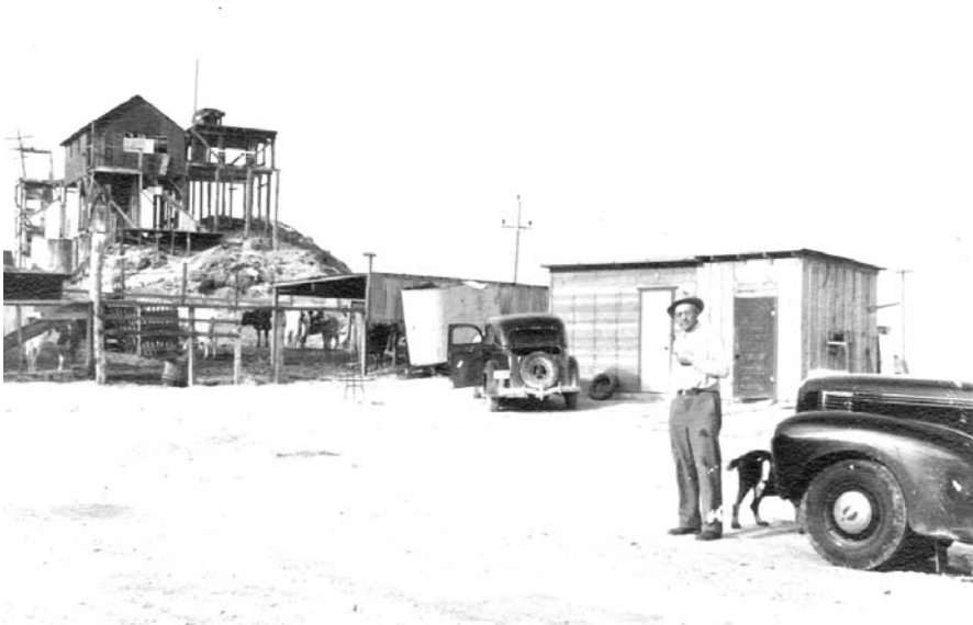
"The dairy was against a small rise, and two of the walls of the dairy were dug out from that rock." Lloyd Mount at the dairy in 1942. (Photograph courtesy of Sarah Grable.)
